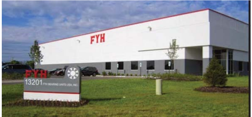
FYH USA will be constructing a 36,800 SF addition to their USA headquarters in Huntley in 2017.
